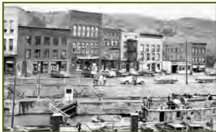
Whitehall's Main Street Historic District, shown here in 1973, remains largely intact and is the focus of the village's continuing community and heritage development activities.
