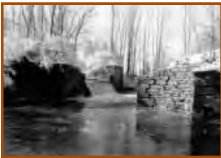
East side of aqueduct.
